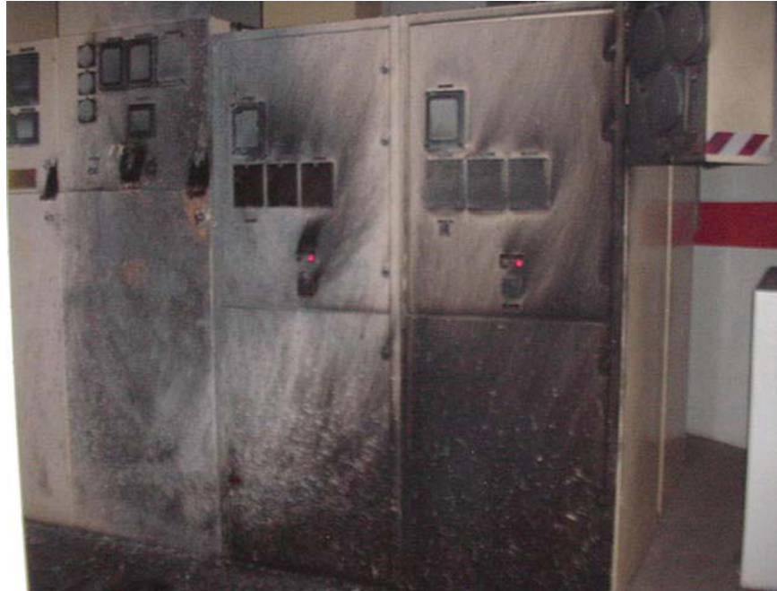
Figure 7-2 Photograph of the surface damage and burning. The photograph shows damage observed for the more heavily impacted cabinets on one side of the aisle-way below the fault point (the cabinet to the left as seen in Figure 7-1).
