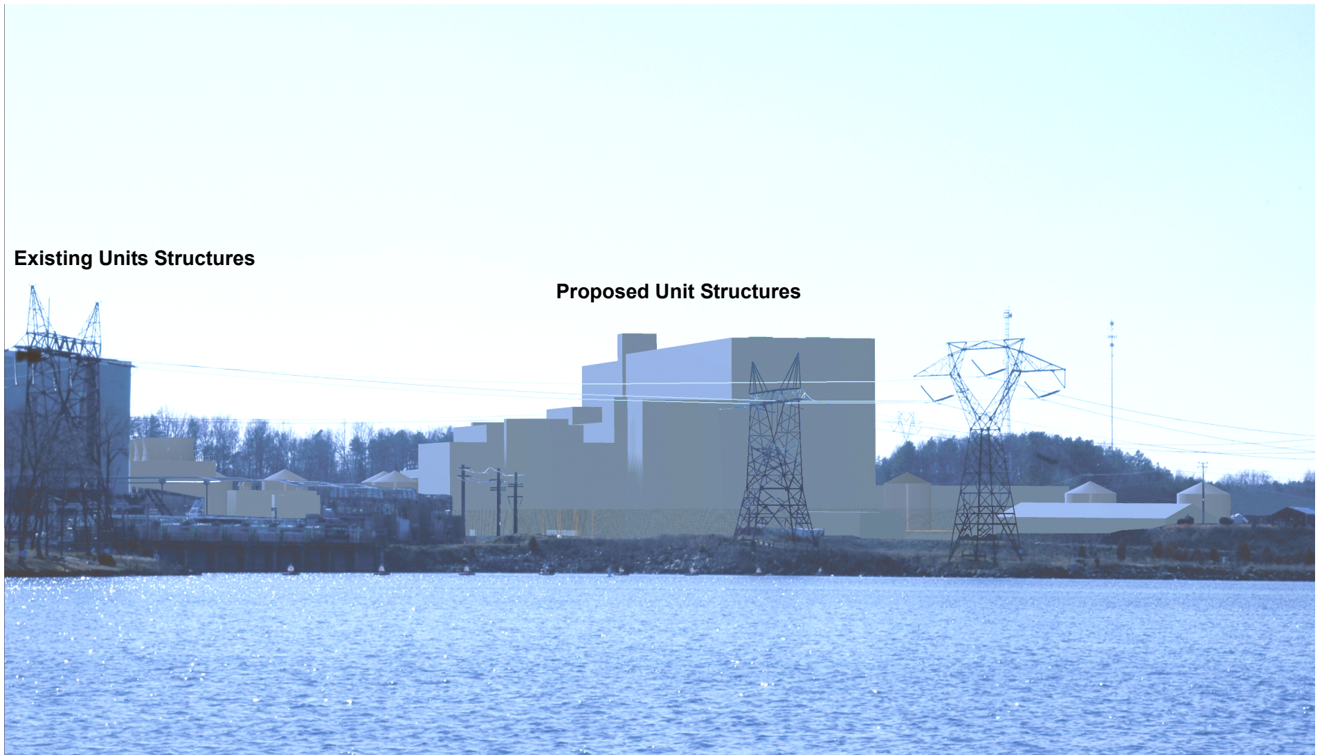
Figure 5.8-3 Looking Southwest from Unit 1 and 2 Intake Area
