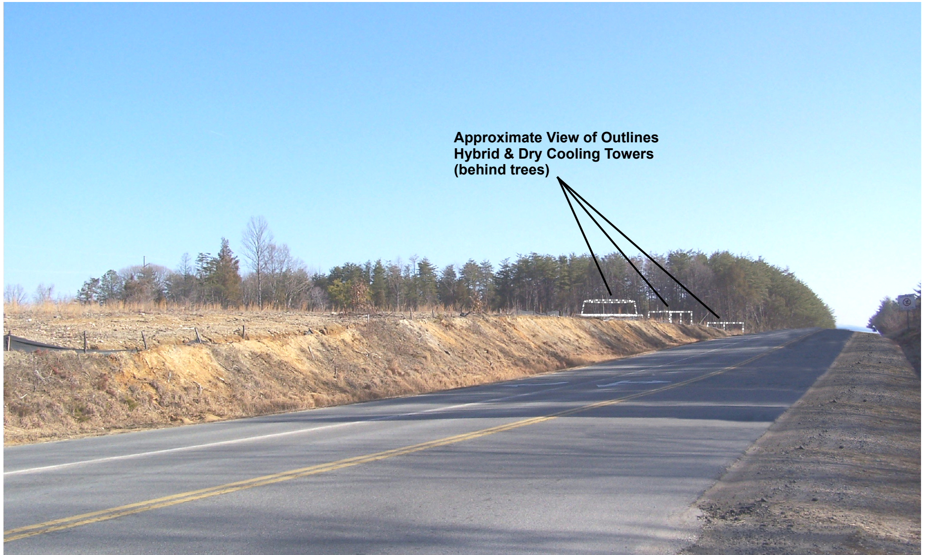
Figure 5.8-1 Looking Northeast Along the Plant Access Road
