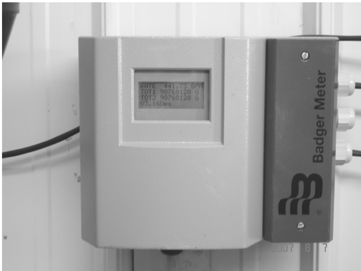
Figure 2.3-3. Computerized Meter for Monitoring Well Field Flow Rates
