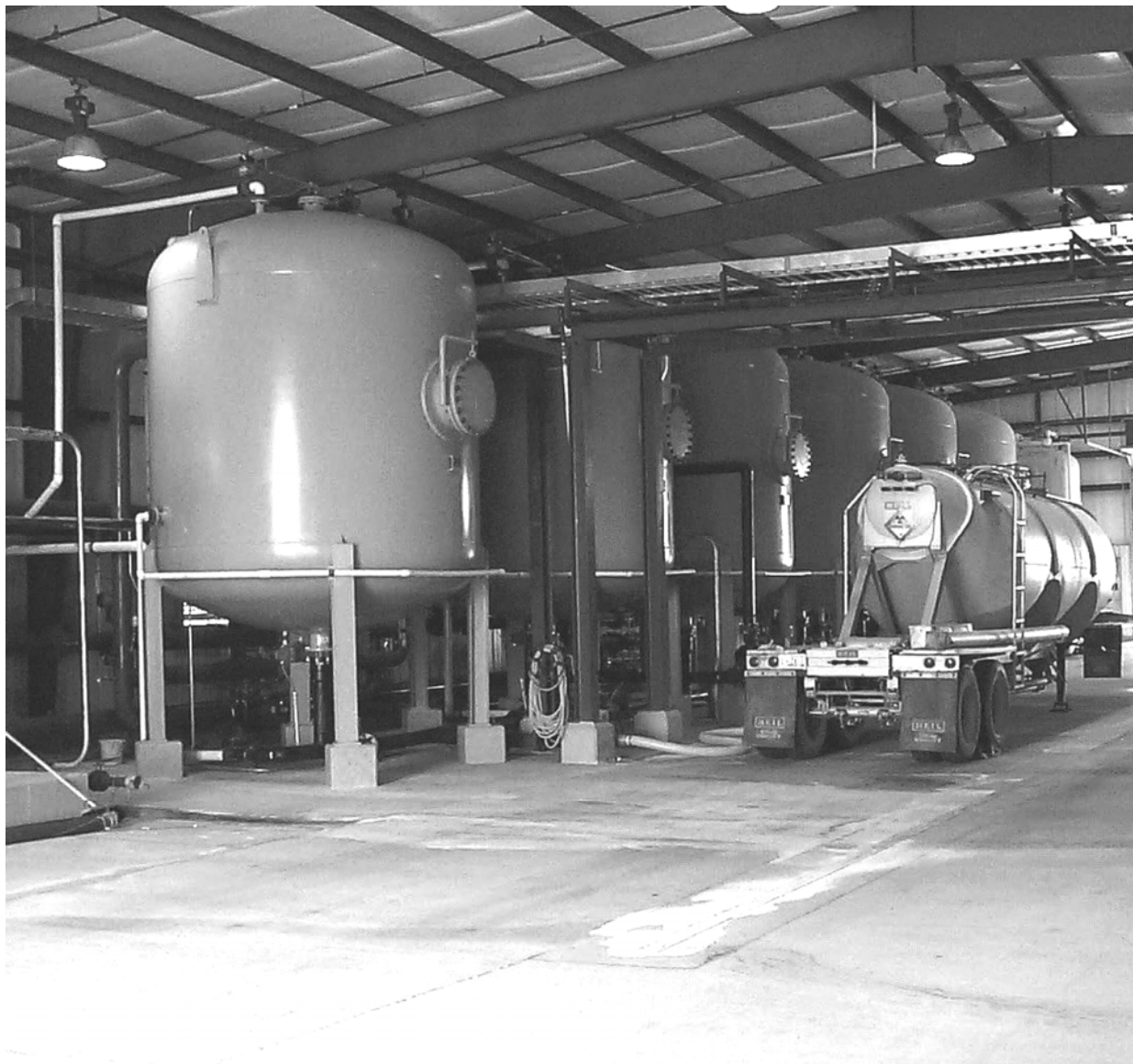
Figure 2.4-3. Typical Ion-Exchange Vessels in an ISL Facility
