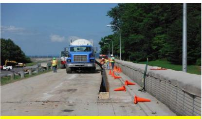
Placement of Flow Fill in Seepage Cutoff for RCC
