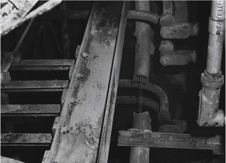
*Picture of Browns Ferry Fire Cable Spreading Room. Note the melted aluminum electrical cable conduit.*
