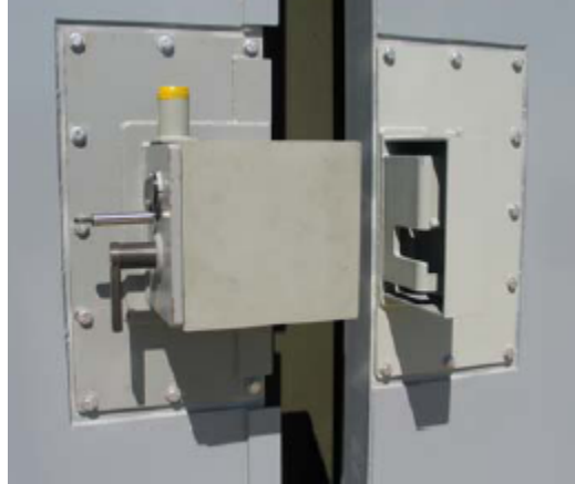
Figure 4. Internal locking device
