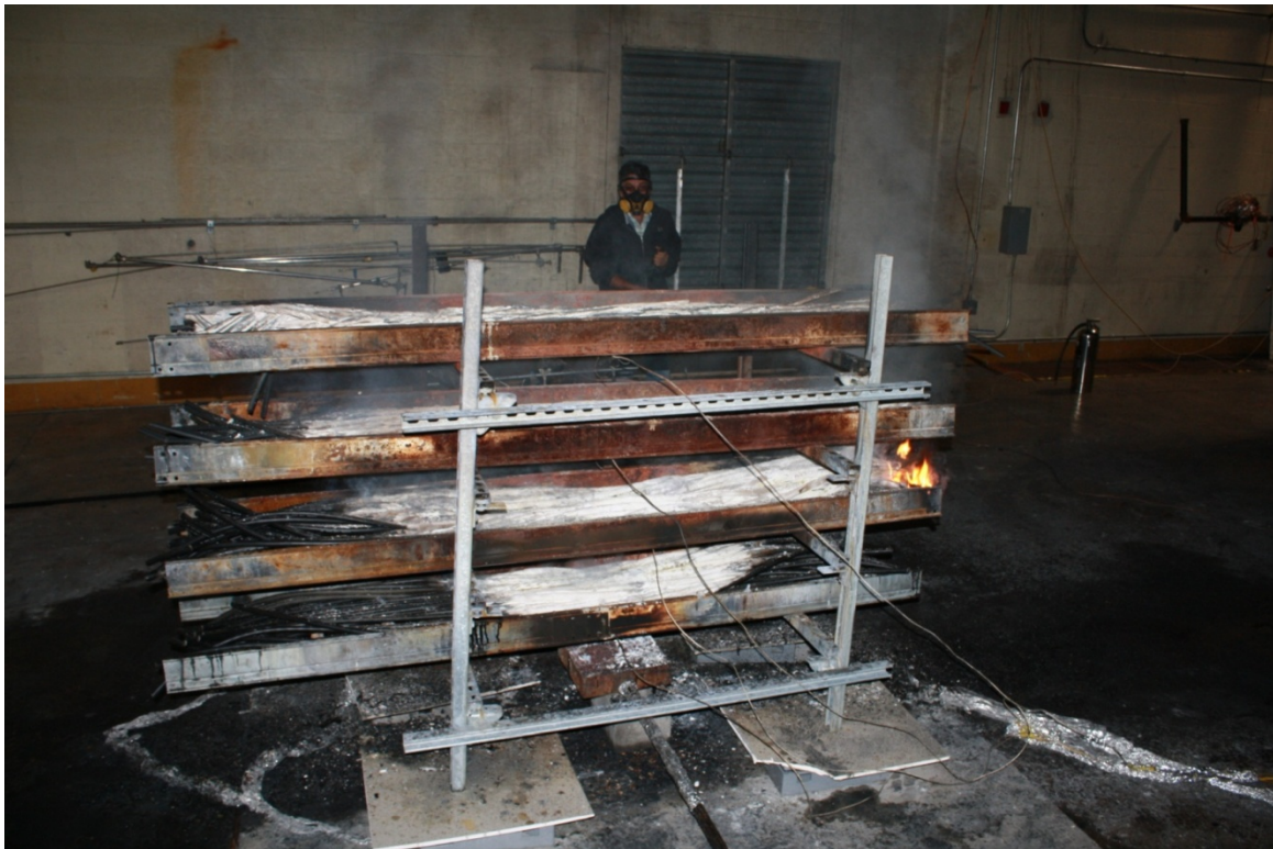
Figure 8-15. Damage to cables following Multiple Tray Test 14.
