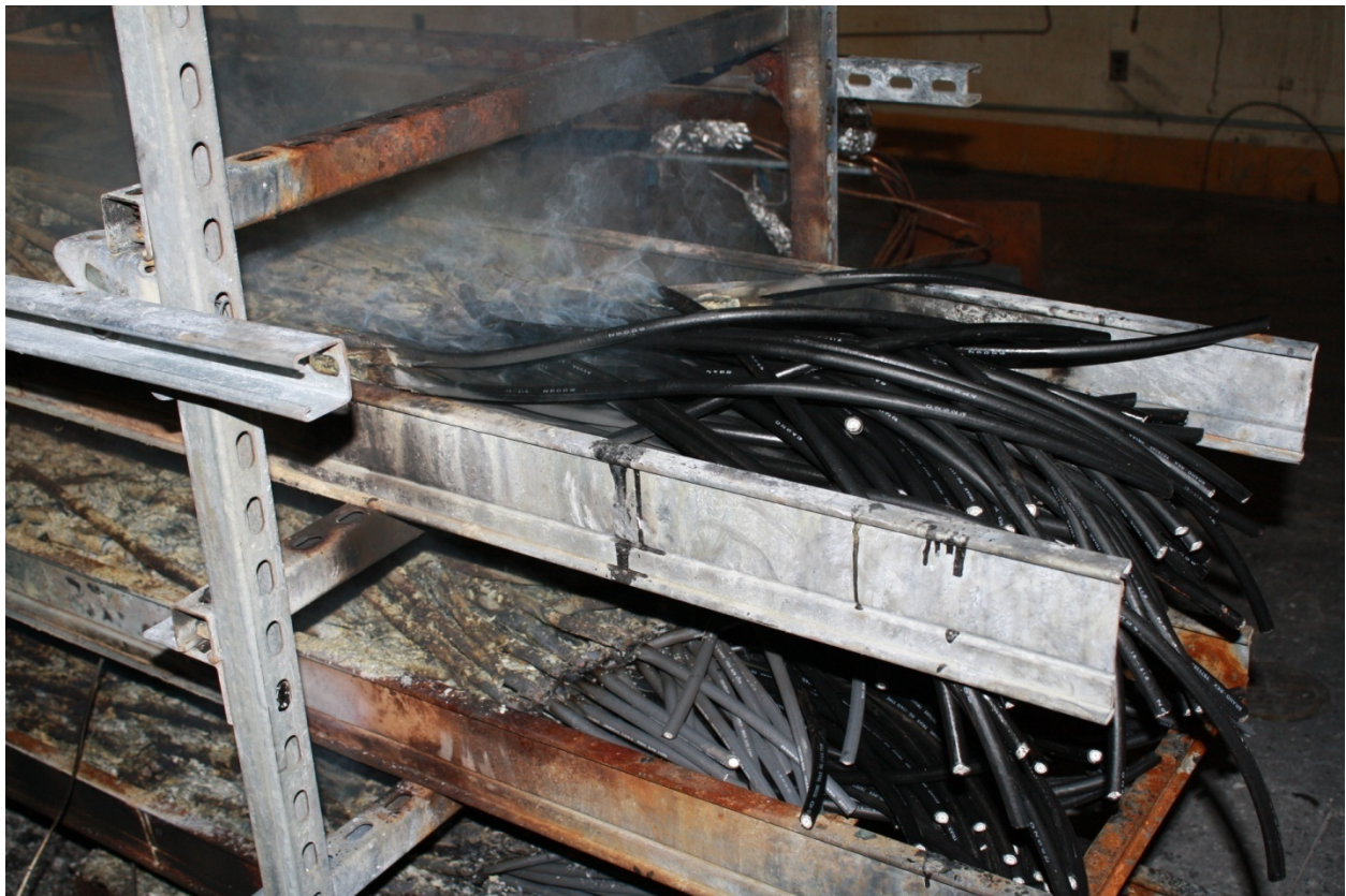
Figure 8-19. Damage to cables, Multiple Tray Test 16.
