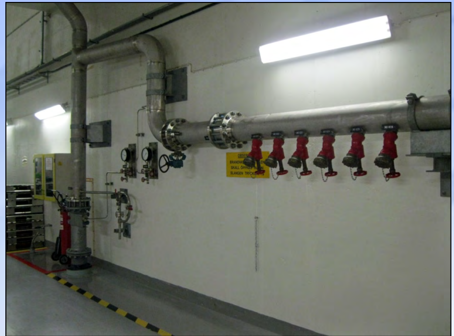
Containment Flooding System Temporary Equipment Connections.
