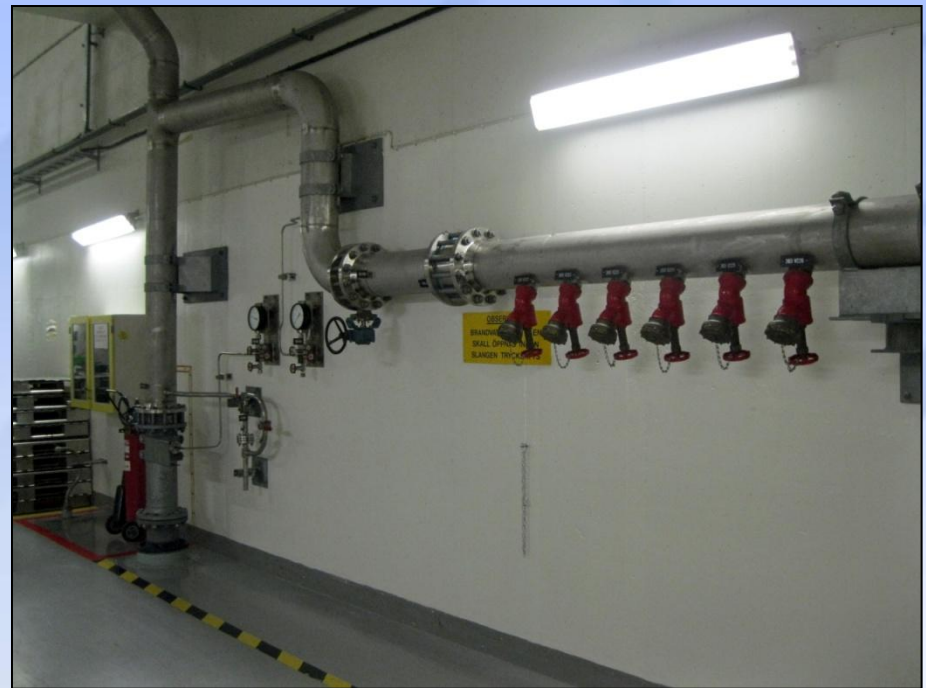
Containment Flooding System Temporary Equipment Connections.
