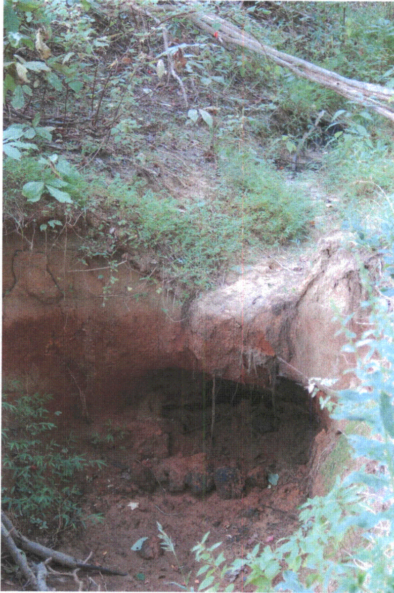
PHOTO 6: Existing head-cut location (proposed step pool location)
