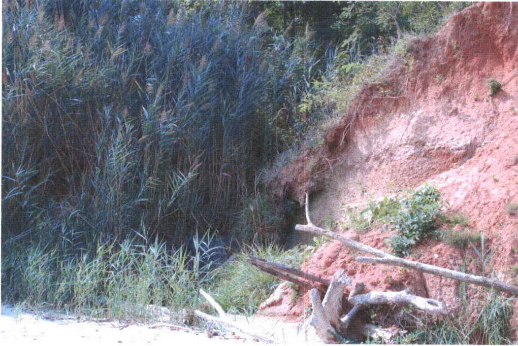
PHOTO 3: Outfall of SE-4 to the Chesapeake Bay
