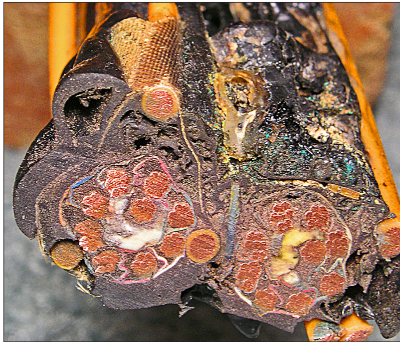
Electrical Cable Fire Damage
