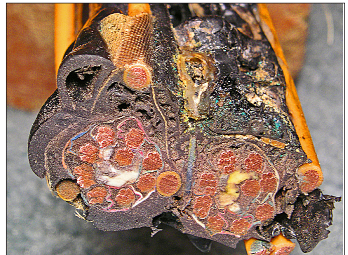
Figure 2.4 Electrical cable fire damage
