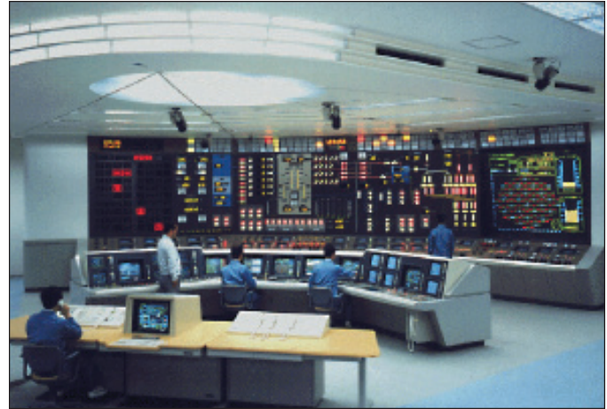
Figure 1.1 Highly integrated control room
