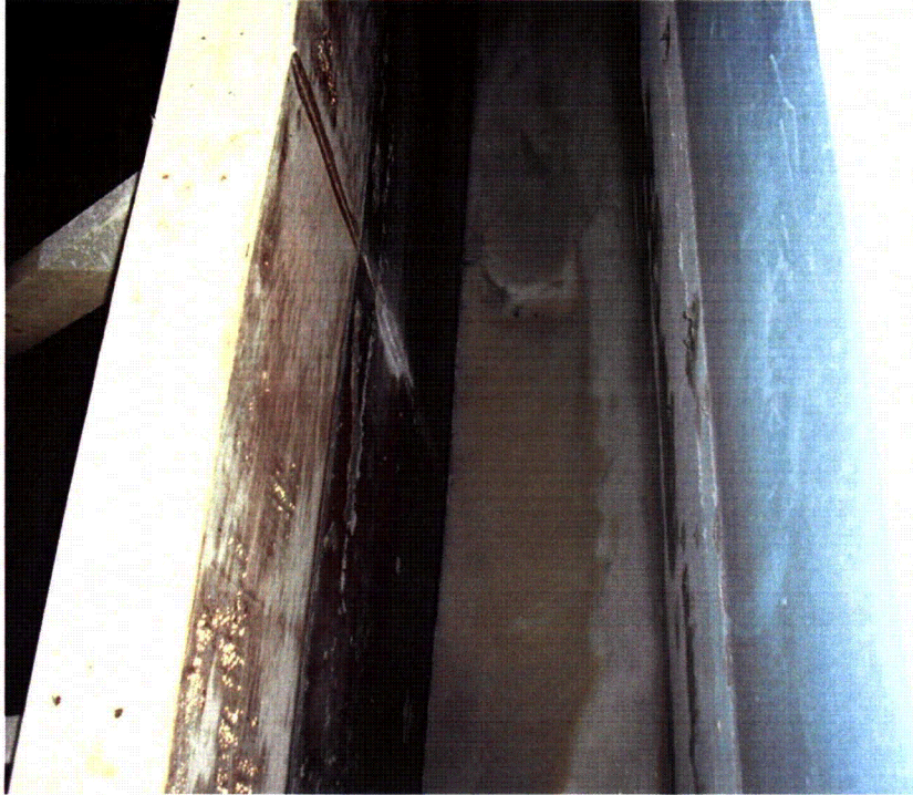
Figure 17-1 Debris Settled On Test Flume Floor During Drain Down
