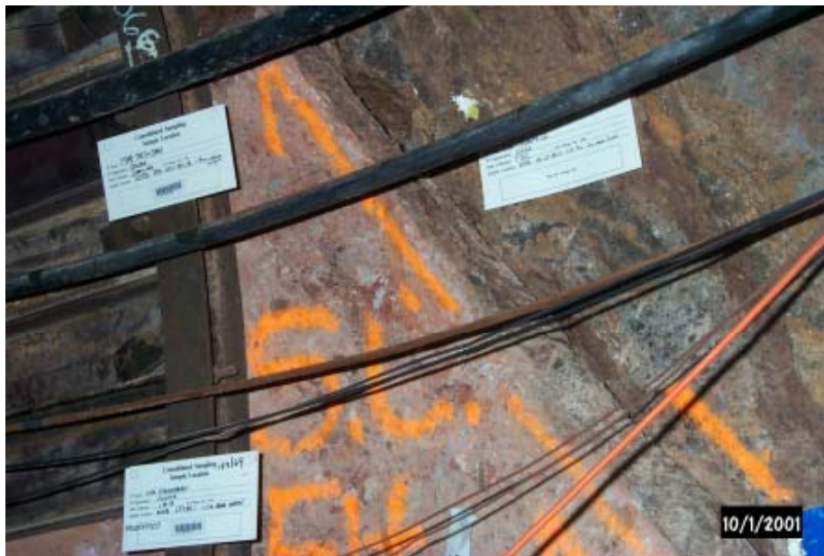
Figure 6-118. Condensate on Shotcrete after Second Bulkhead
