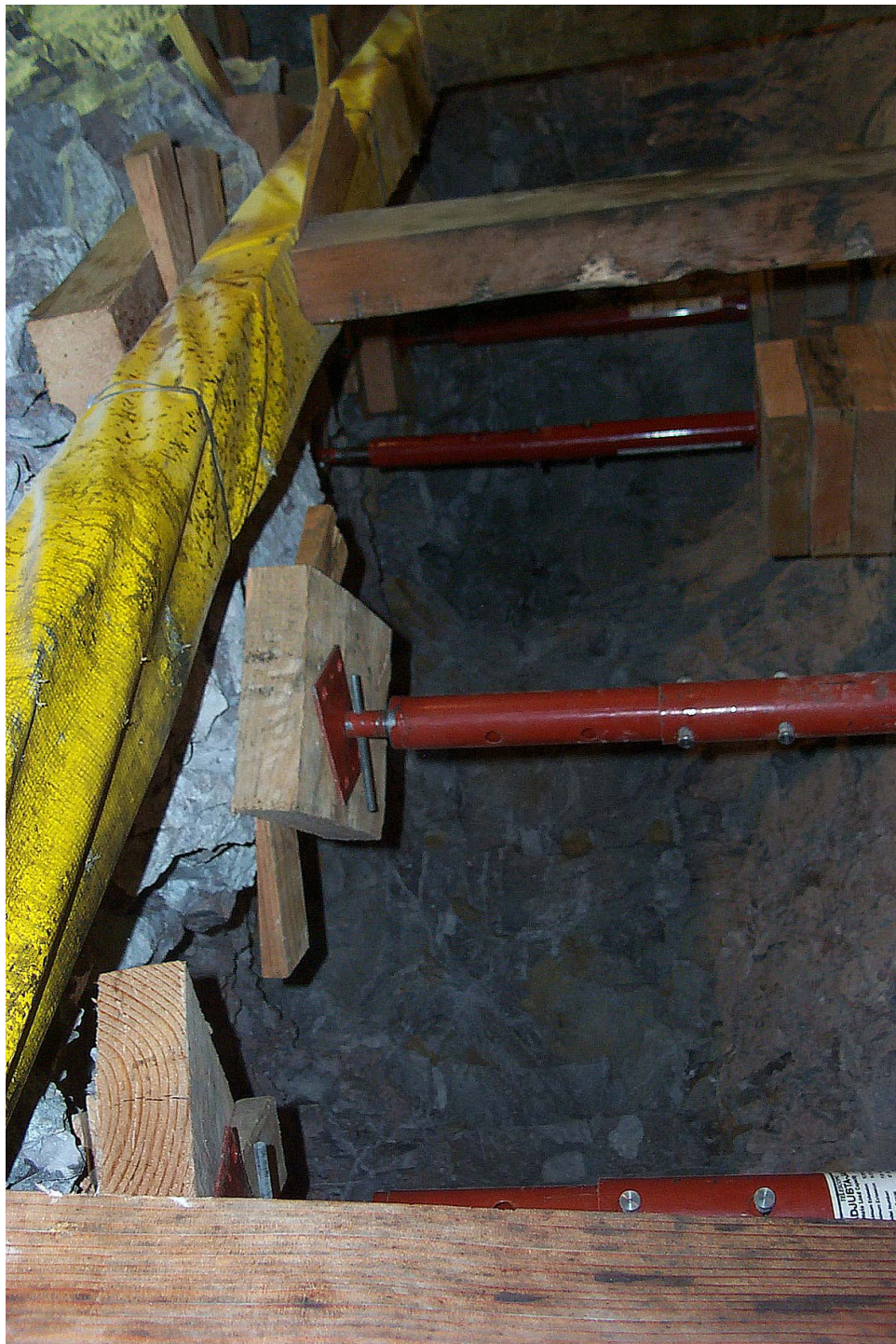
Figure 6-38. Photograph of Left (East) Rib of Niche 5 (Niche CD 1620) Showing Ceiling of Slot and Ground Support
