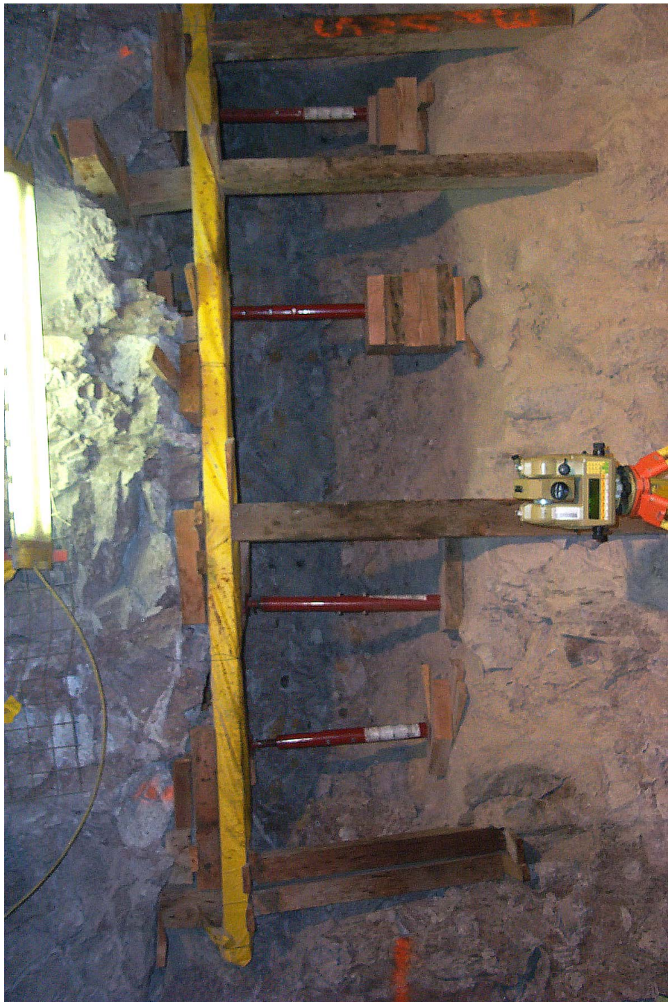
Figure 6-37. Photograph of Left (East) Rib of Niche 5 (Niche CD 1620) Facing the Opening of a 3.3-m-Long Slot and Showing Ground Support
