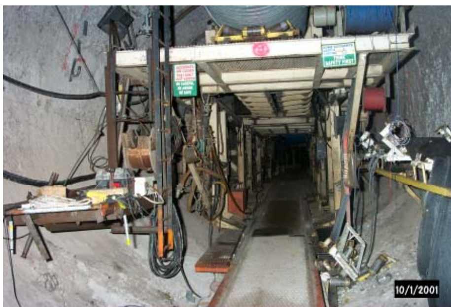
Figure 6-120. Tarp Discoloration before CD 25+99 Bulkhead
