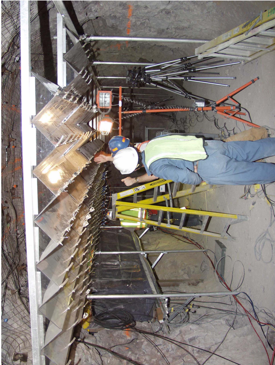
Figure 6-40. Capture System Installation Showing Plastic Capture Trays and Tarp in Slot
