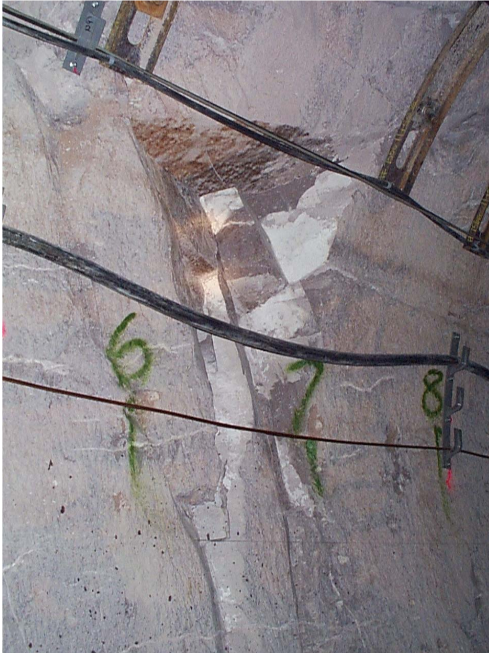
Figure 6-14. Evidence of Key-Block Occurrence in the ECRB Cross-Drift, Station 11+55
