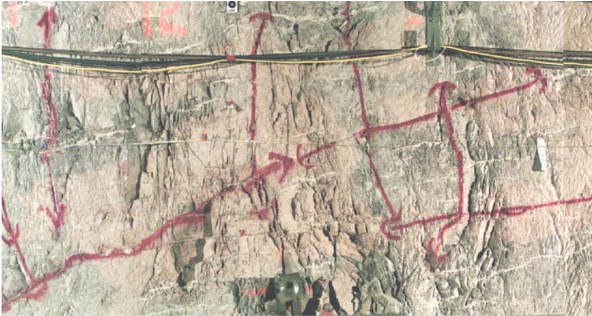
Figure 6-8. Fractures in Wall of the ECRB Cross-Drift in the Ttpmnn
