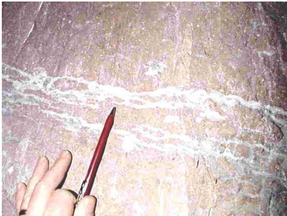
Figure 6-9. Low-Angle Vapor-Phase Partings in Nonlithophysal Units in the ESF
