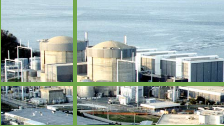
Calvert Cliffs Nuclear Power Plant, Lusby, Maryland.
