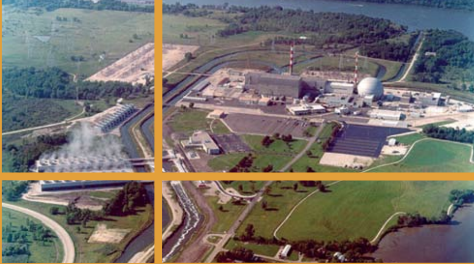
Dresden Nuclear Power Plant, Warrenville, Illinois.
