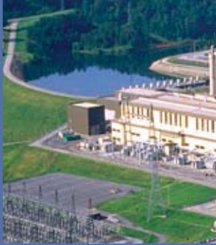
Oconee Nuclear Power Plant, Seneca, South Carolina.
