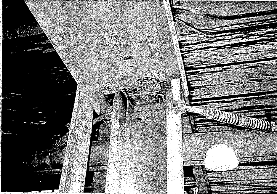
Item 34 - Unit 2 Elev 960 Front Boiler Buckstays Bent - Plate 1
