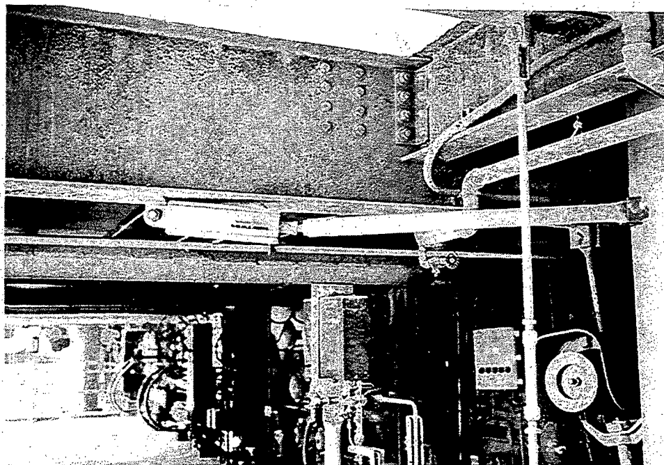
Item 45 - Unit 4 Elev 945 Hot Reheat Steam Line Snubber by Fuel Oil Differential Pumps Bent
