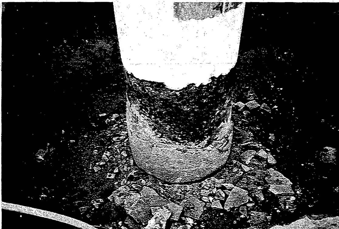
Glendale: Picture 35 (20" Vertical Riser to Cooling Tower Damage)
