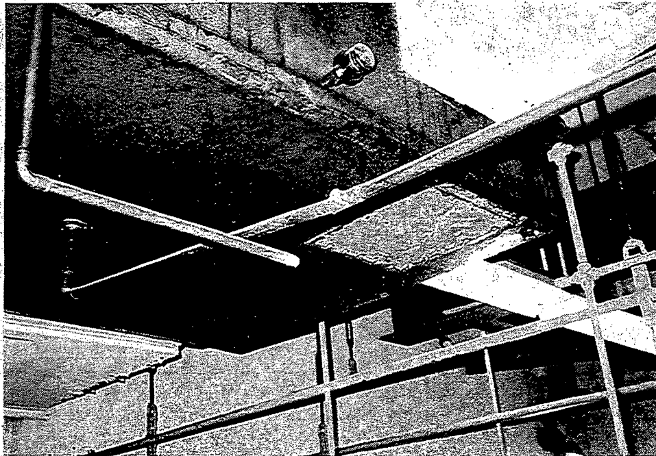
Item 62 - Unit 1 & 2 Elev 992 Column G9 Condensate Drain to Air Conditioner in Chem Feed Room Broken
