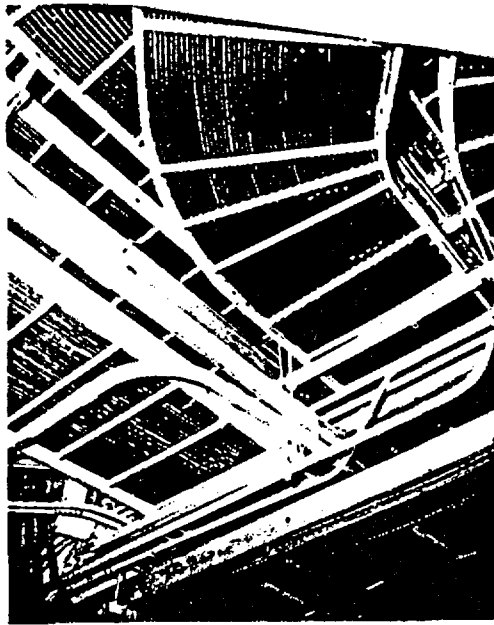
FIGURE X A-49 Electric Power and Control Cables Installed in Cable Trays
