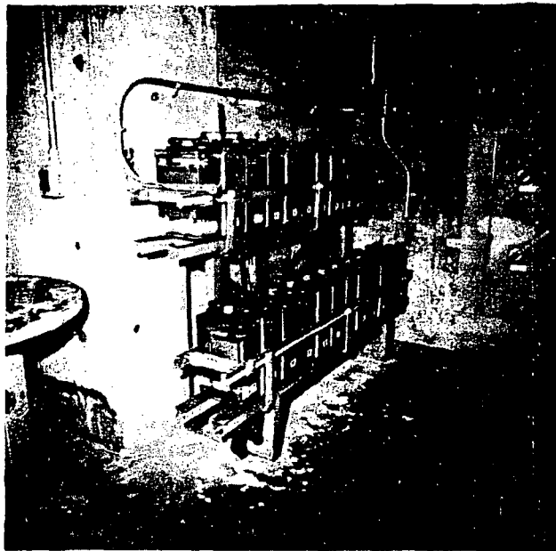
FIGURE X A-47 Batteries and Battery Racks - 24-V System
