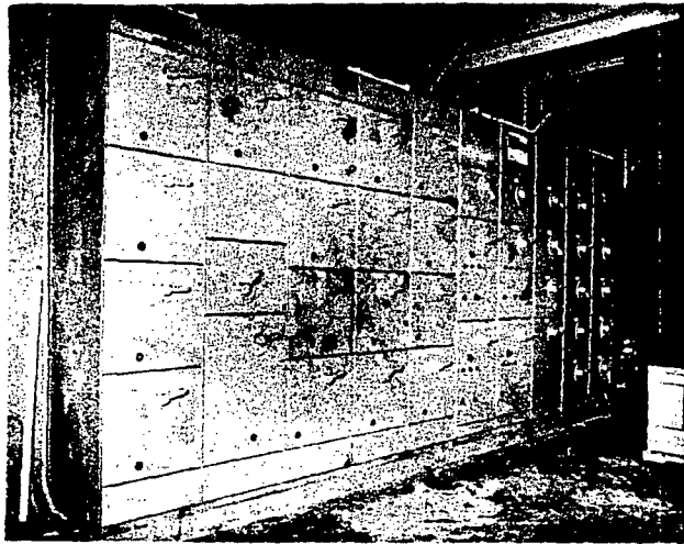
FIGURE X A-53 480-V Motor Control Centers
