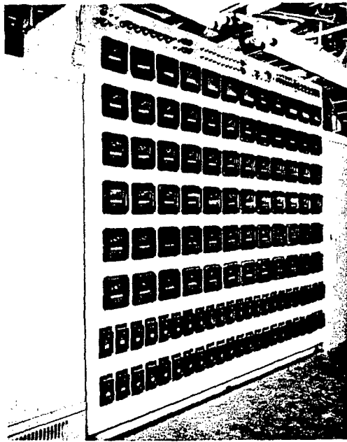
FIGURE X A-57 Reactor Protection System Logic Cabinet
