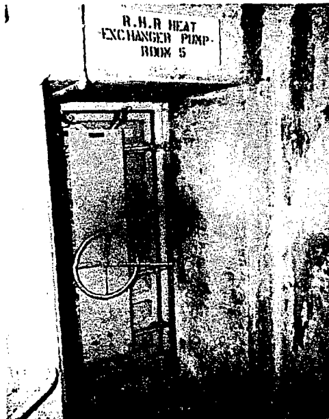
FIGURE X A-36 Watertight Entryway to RHR Pump Room
