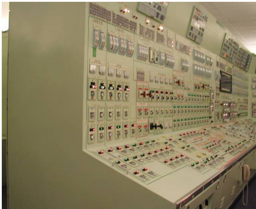
Figure G-20 Example of a Main Control Board
