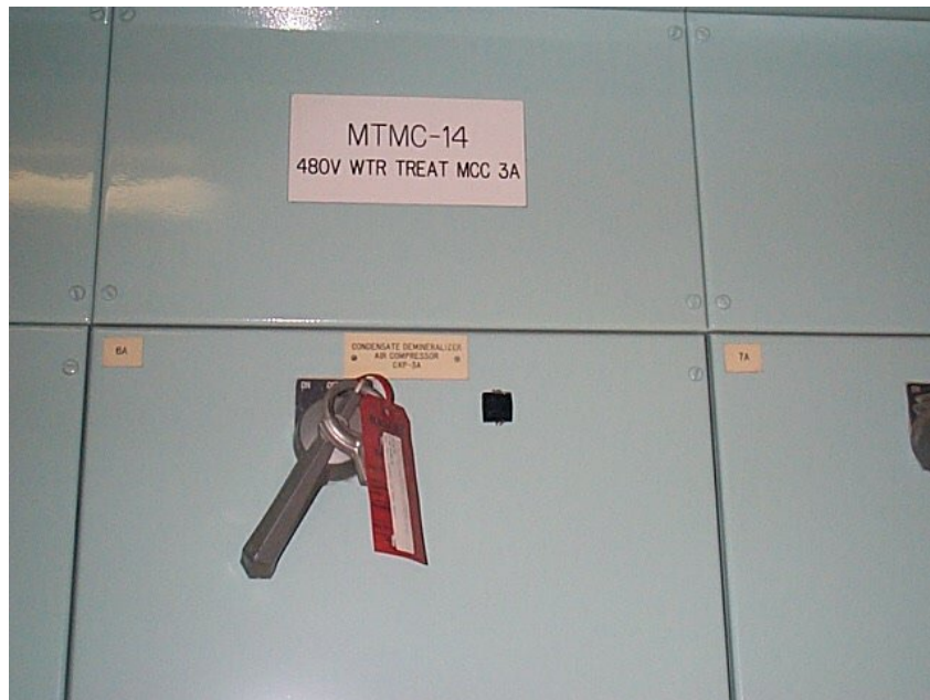
Figure G-6 480 V Switchgear (Front)
