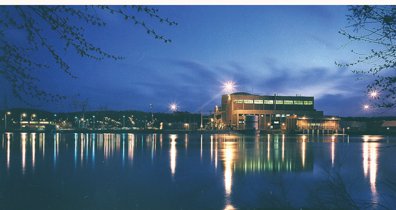
Fort Calhoun Nuclear Power Station
