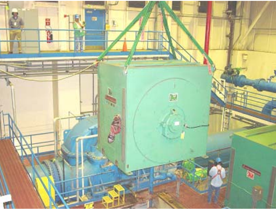
#1 Circulating Water Pump Motor
